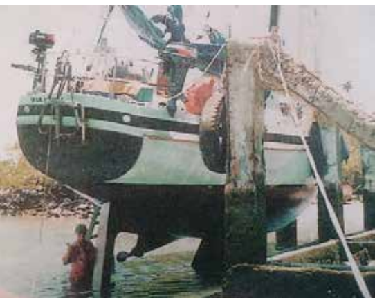
Repairs at Galapagos.
